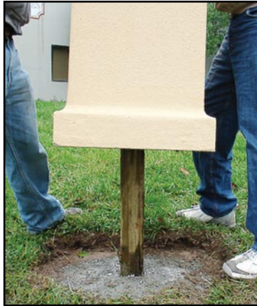
Column is easy to install over your 4" x 4" wood post.
